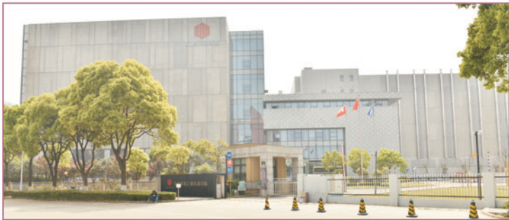
Shanghai Data Center
