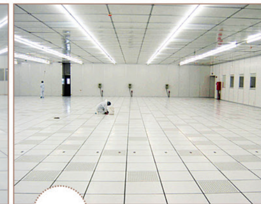
10K class clean room
