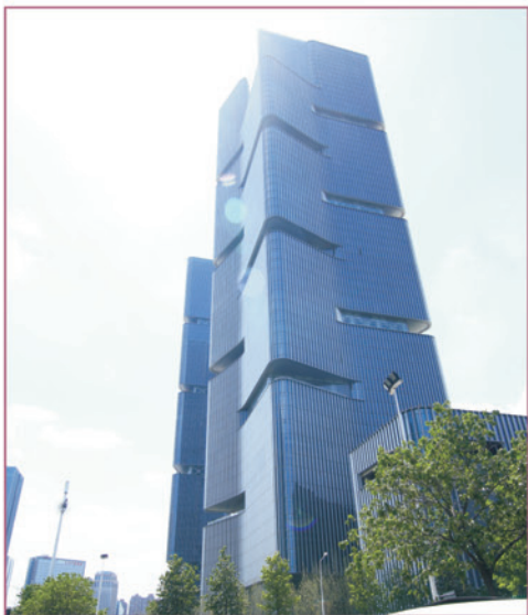
Zhengzhou greenland Center
